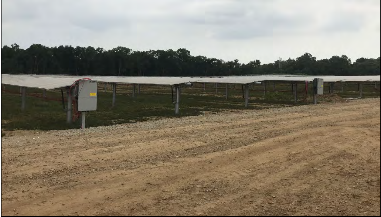
Inset 4. Access road along solar array (Photo: Open Road Renewables).
