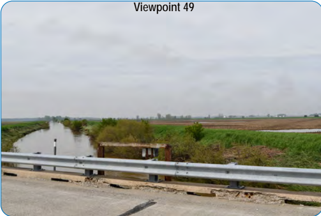
VP 49 | View looking West from County Road 20 and Bean Creek in the Township of Gorham, Fulton County.
