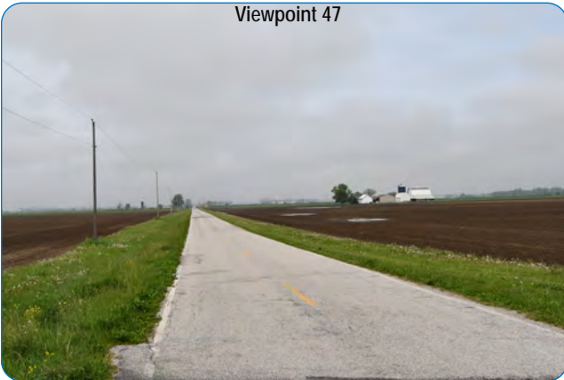
VP 47 | View looking West from County Road N in the Township of Gorham, Fulton County.
